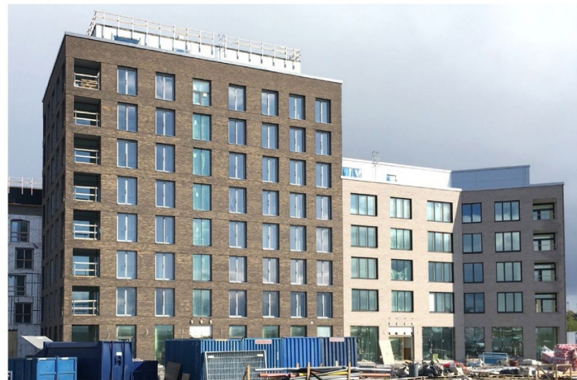
Herttuankulma, Lundén Architecture Company/ FI
