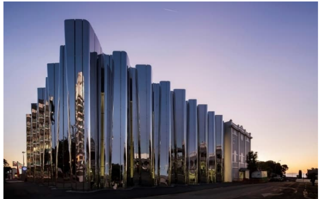
Len Lye Center, Patterson Architects
