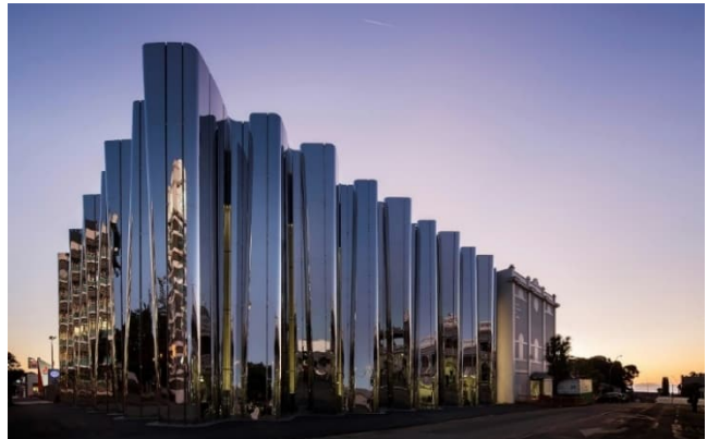
Len Lye Center, Patterson Architects
