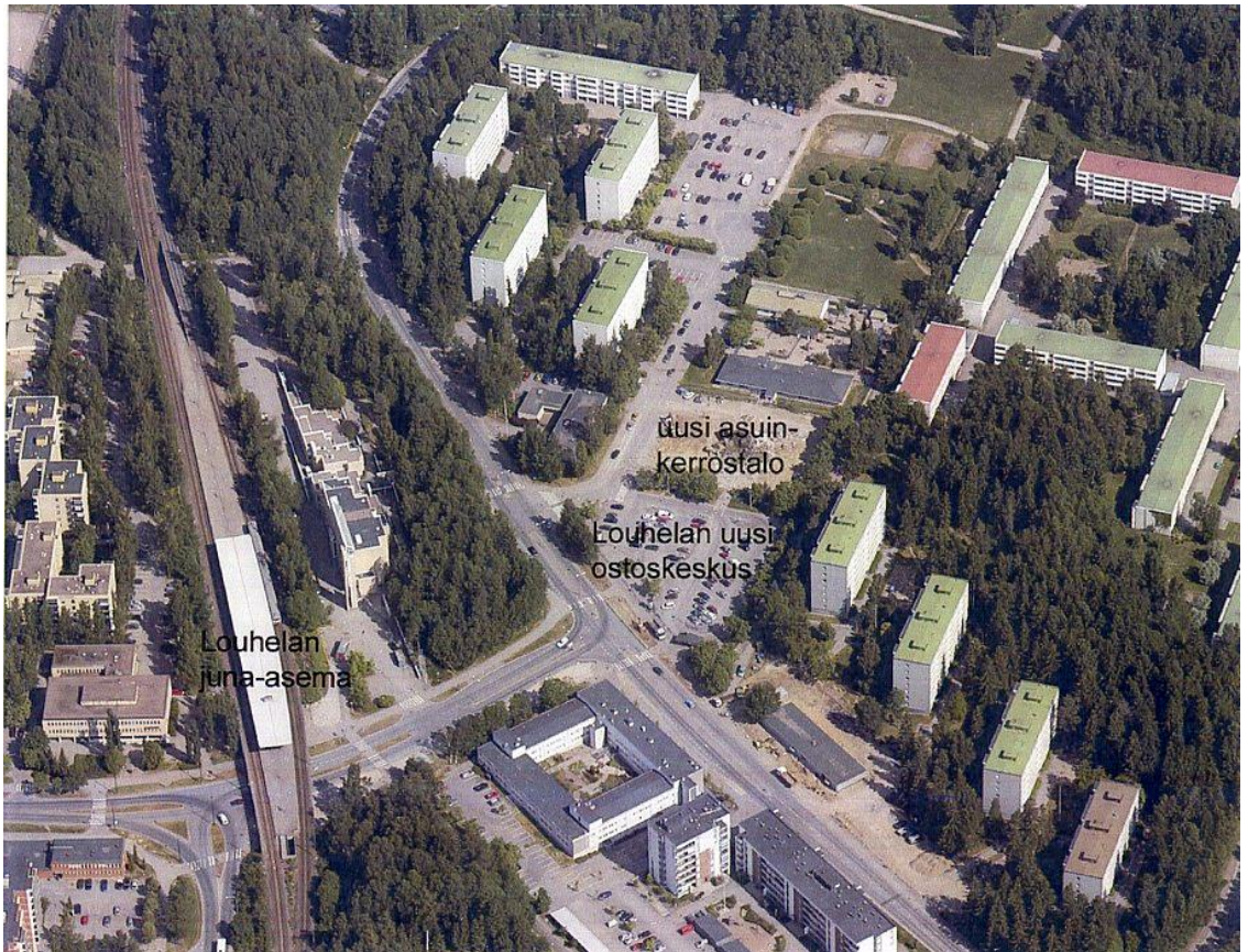
Louhela urban development area. Aerial photograph (2011) showing the new shopping center and apartment building.
